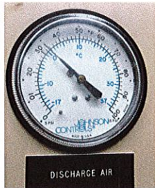
Broken discharge air temperature gauge (reads erroneously)
